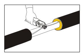
Insert the other wire into the connector and crimp it.
